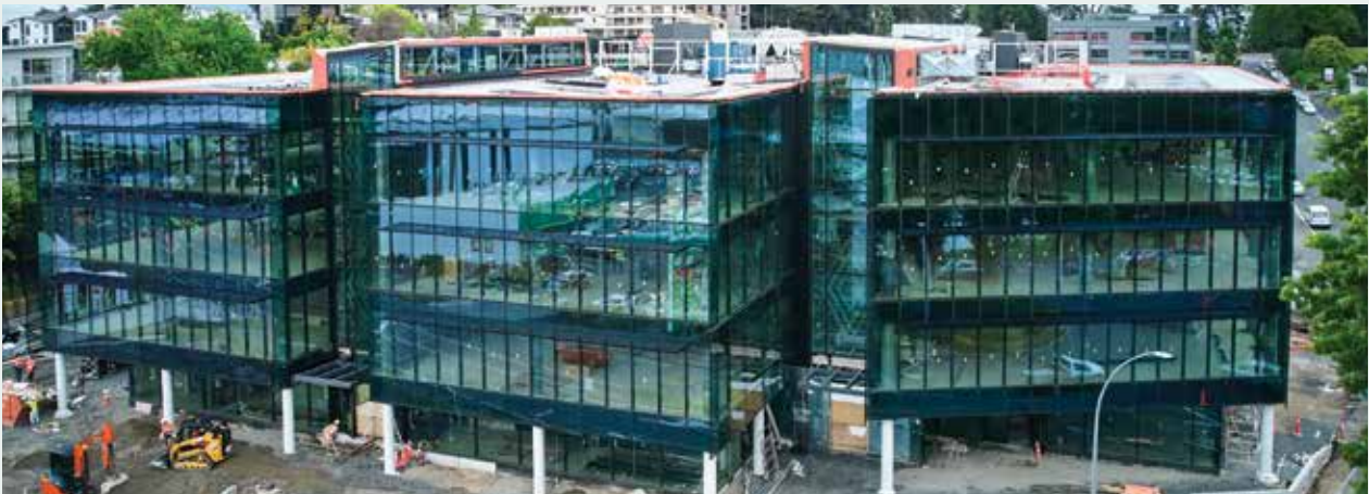
ACC Building progress November 2022.
