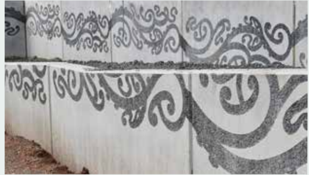
Retaining walls in progress.
